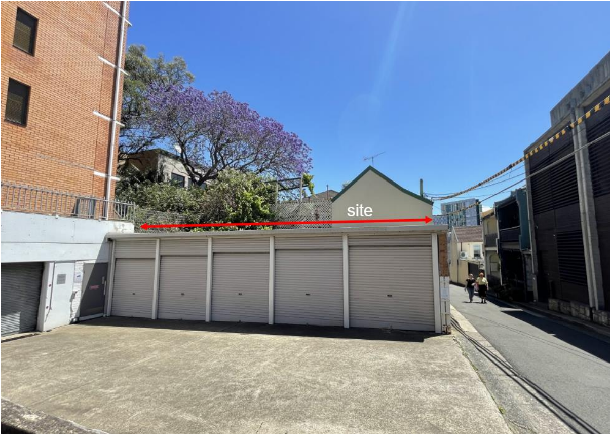
Figure 4: West elevation viewed from Wells Street
