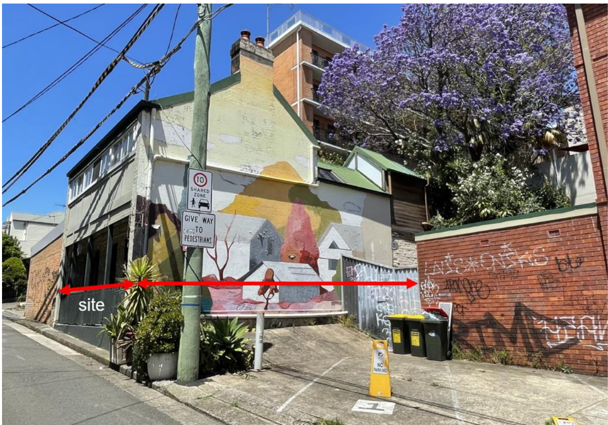
Figure 3: East elevation viewed from Wells Street, showing existing rear addition
